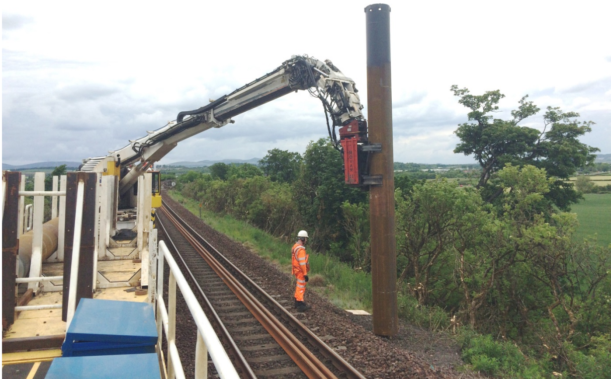
Installation of an 8.0m pile on EGIP.
